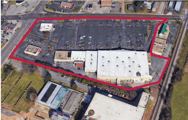
Aerial of the Roses Shopping Center site.
